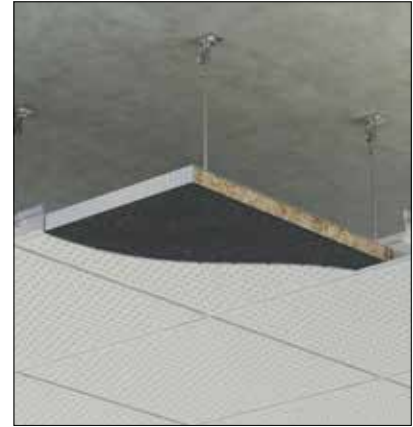
Rockfibre Acoustic Pad MP562 installed in metal grid ceiling system.
